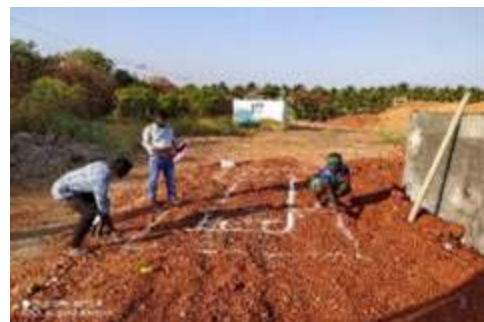
Figure 3.2: Marking of Screen Chamber
