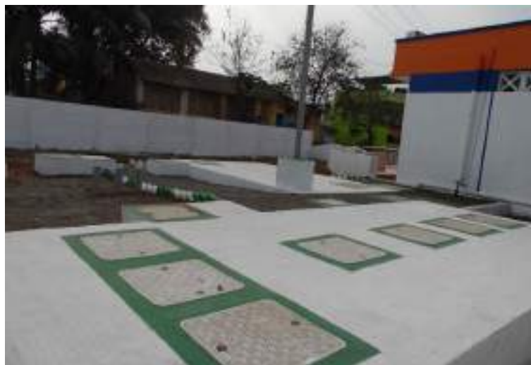
Figure 6.5: Improved Septic Tank After Construction
