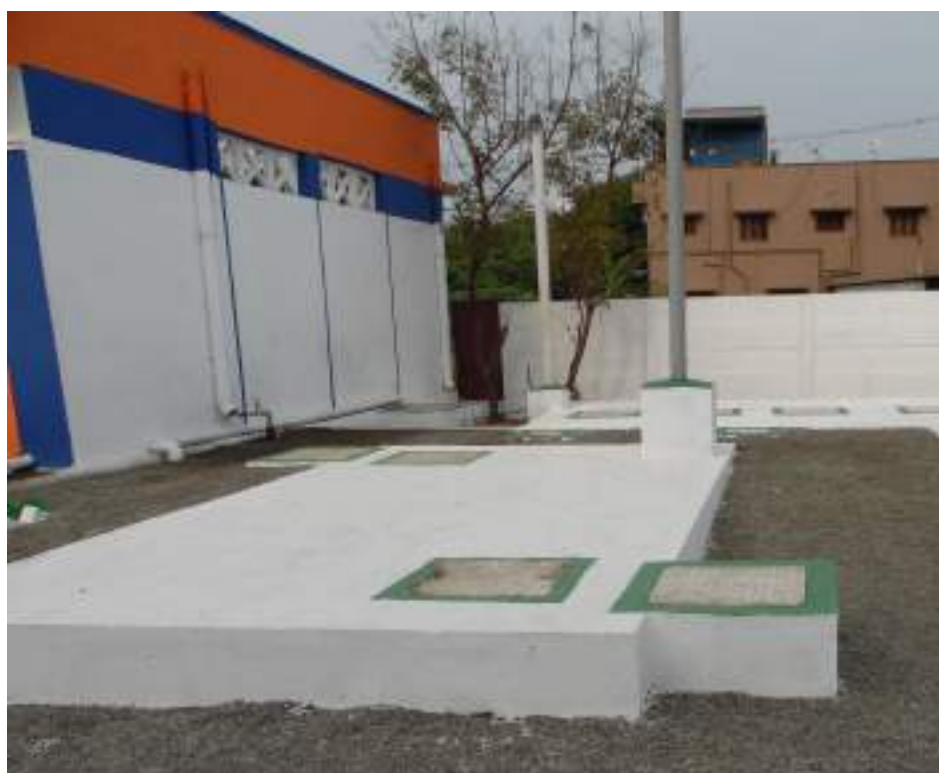
Figure 6.2: Primary Settler After Construction
