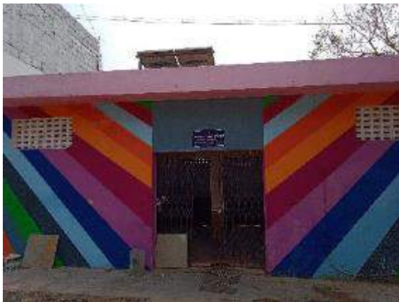
Figure 2.4: Toilet at Anna Nedunsalai, Zone 14
