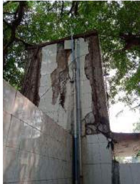
Figure 2.3: Toilet at Guindy Bus Stop, Zone 13
