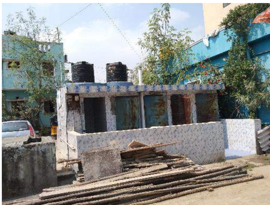
Figure 3.1: Lack of Separate Entrance for Women, Mylai Balaji Nagar CT, Zone 14
