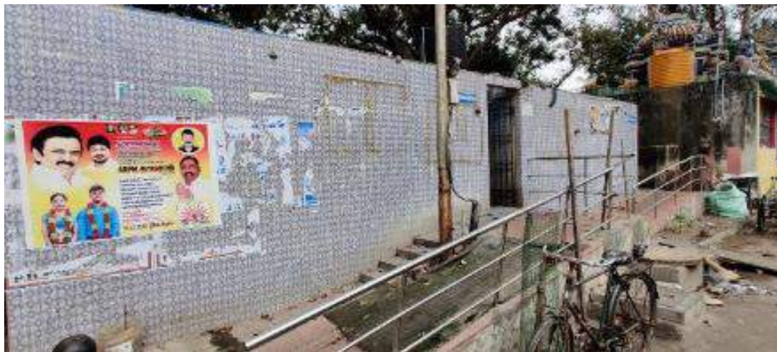
Figure 3.2: Toilet for the Physically Challenged at Rajiv Gandhi Nagar CT, Zone 5
