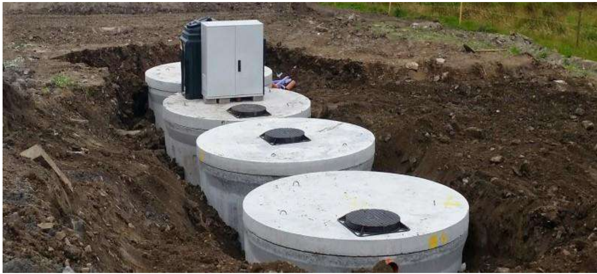
Figure 7.3: Septic Tank Riser
