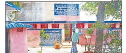
FOR PUBLIC GOOD: A community toilet at Viragupettai in Trichy
