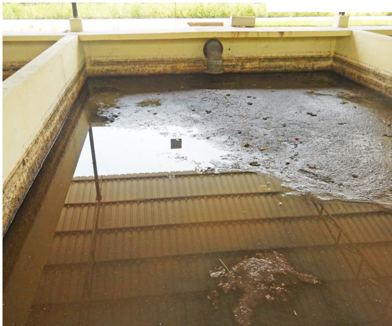
A close-up view of the Sludge Drying Beds
