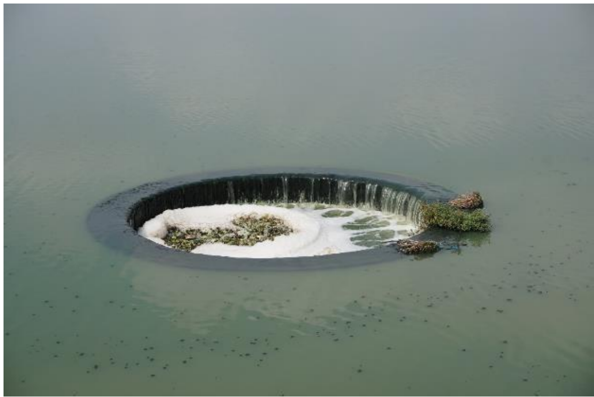
Figure 2.14: Facultative pond outlet structure
