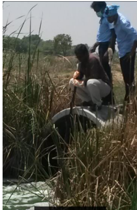
Figure 2.17: Discharge Pipe for Final Effluent
