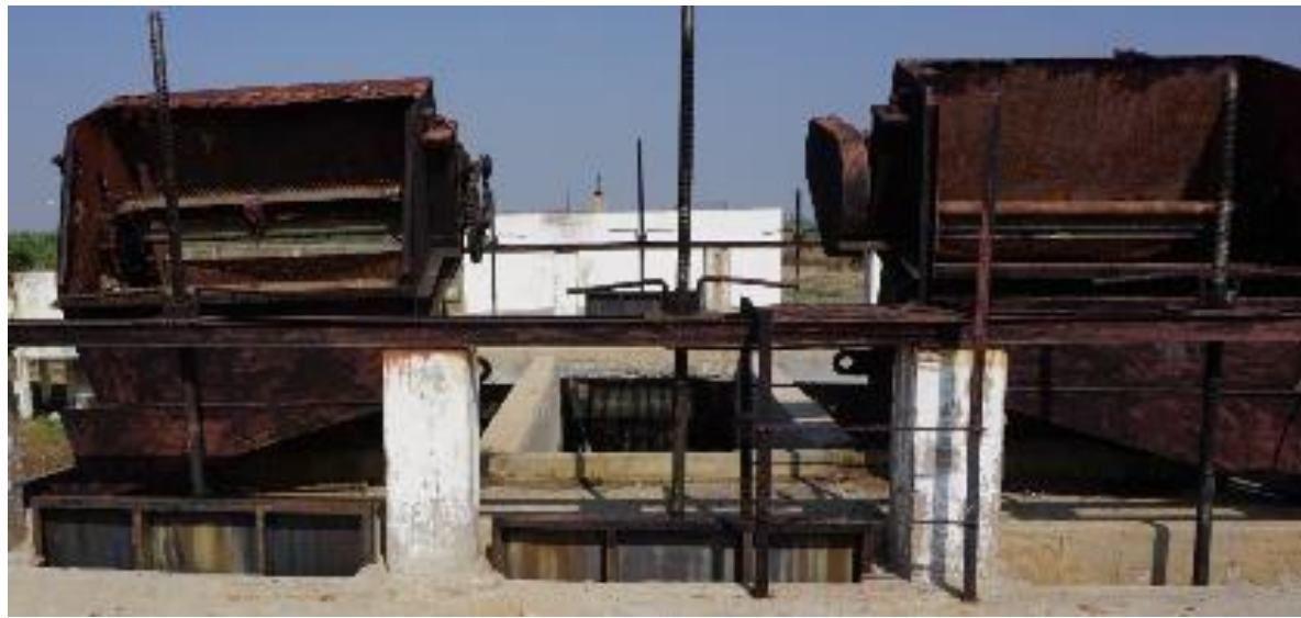
Figure 2.6: Screening system at head works
