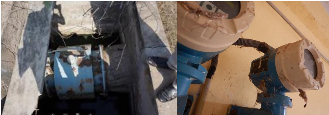
Figure 2.5: Electromagnetic Flowmeter
