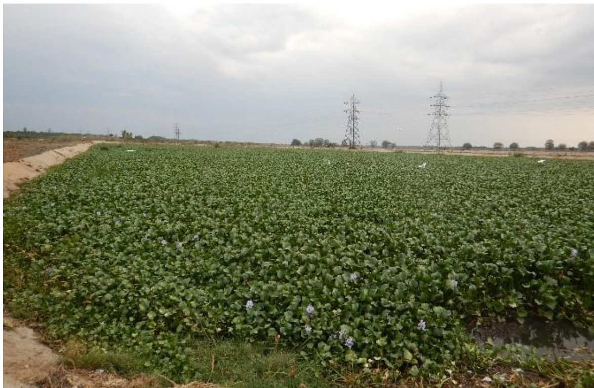
Figure 2.9: Anaerobic Pond with Surface vegetation
