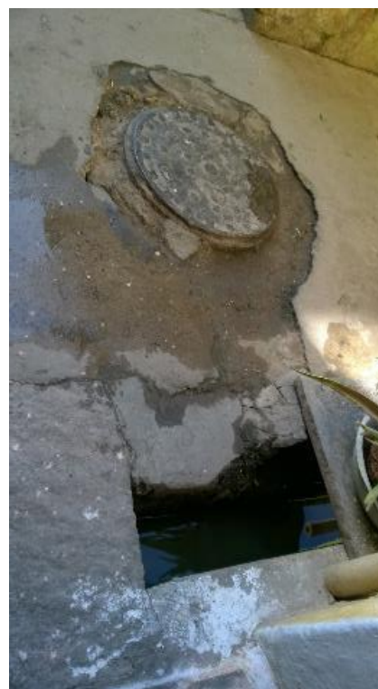
Figure 4.10: UGD By-Passed Resulting in SWD Flows
