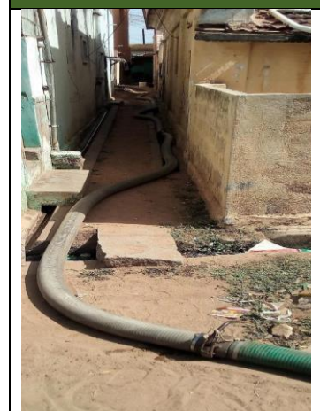
Figure 3.3: Narrow Lane De-sludging at E. Pudhur
