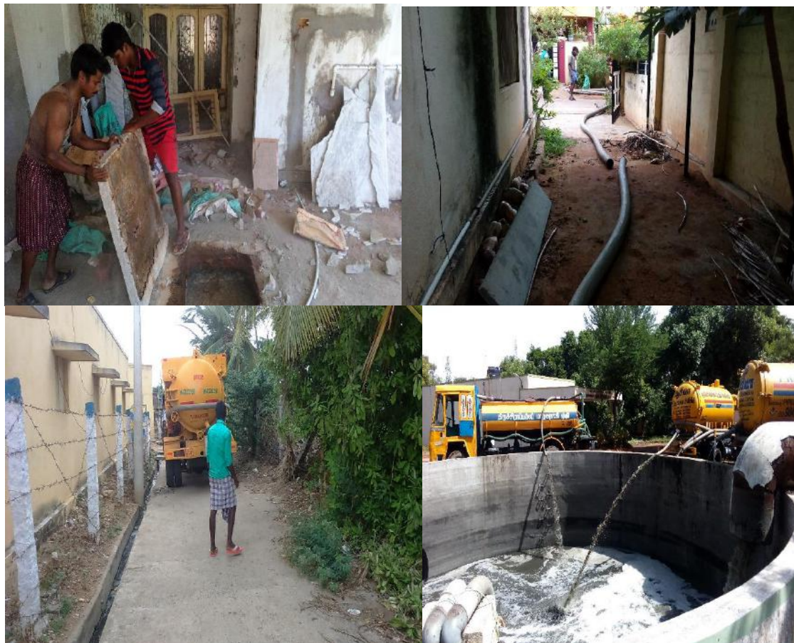
Figure 3.11: Collection and disposal of fecal sludge from households in Tiruchirappalli
