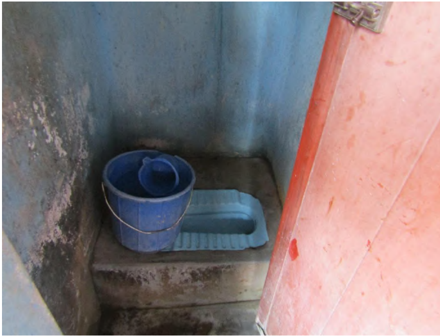
Figure 3.3: Community toilet showing small plinth area
