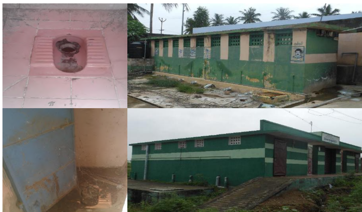
Figure 4.3: Community toilets in Town Panchayats
