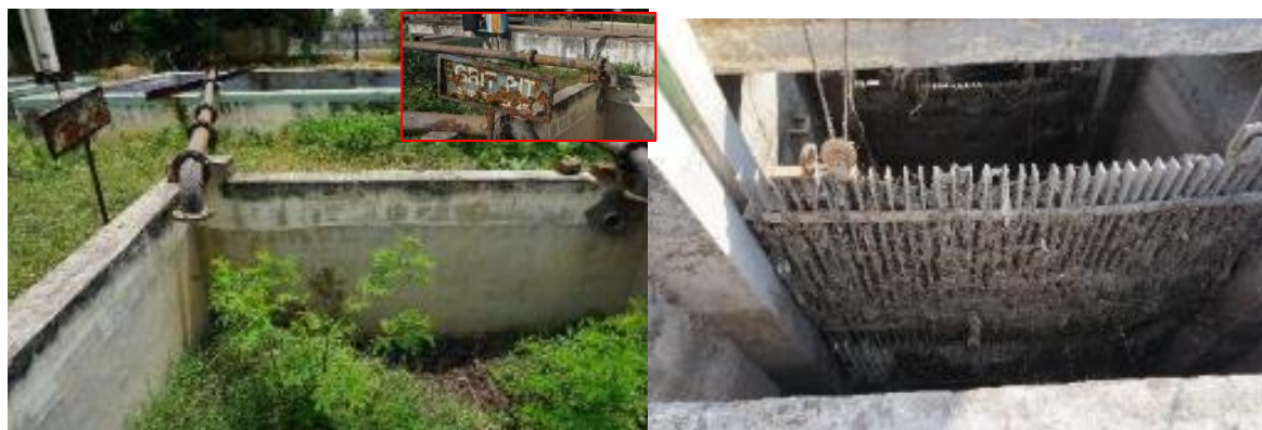
Figure 3.1: Grit Pit and Screening Systems – Not Being Maintained in Anna Stadium
