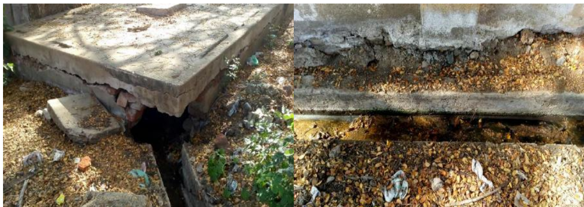
Figure 2.9: Septic Tank Overflow at an FOL in Ariyamangalam Zone Ward 64 – Bhagavathipuram
