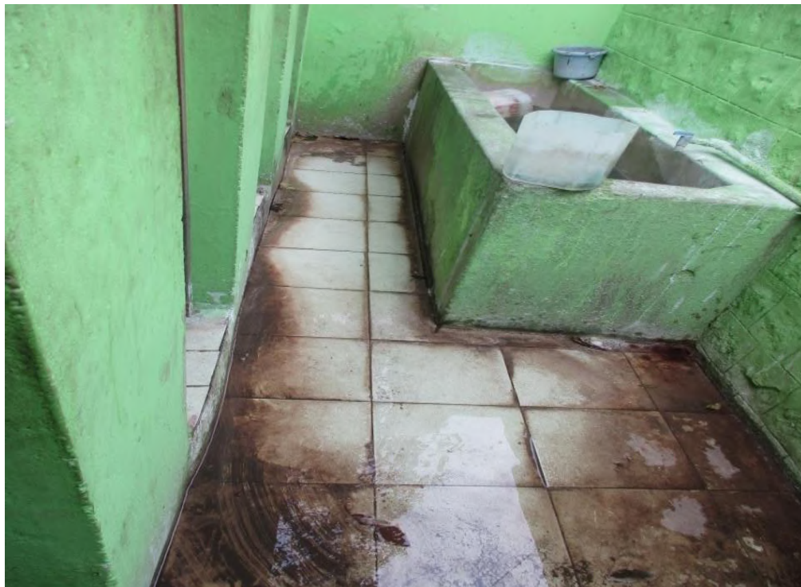
Figure 3.12: Water Storage Tank in a CT
