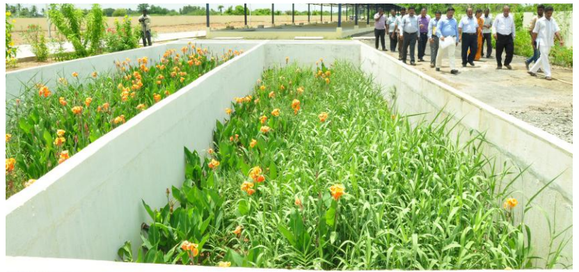
Horizontal Planted Gravel Filter
