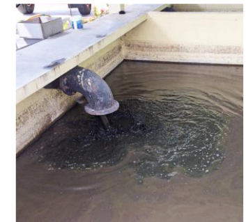
3. FS enters the Sludge Drying Beds (SDBs) & undergoes solid-liquid separation
