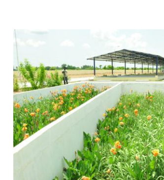
6. The filtrate from the SDBs are conveyed to the Horizontal Planted Gravel Filter (HPGF) reducing the organic matter & nutrients
