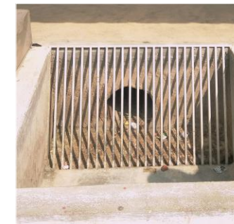
2. Bar screens remove floating debris and other coarse particles
