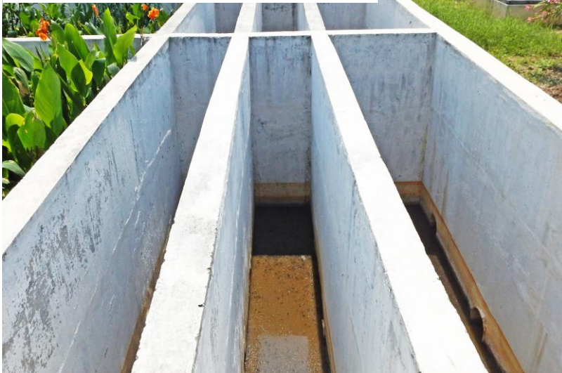
The residual liquid (leachate) passes through stoneware pipes to the Horizontal Planted Gravel Filter
