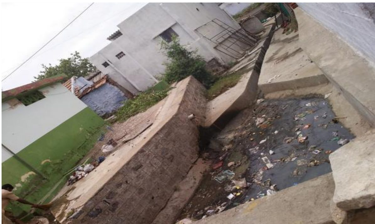
Figure A.8: A view of the open drain in Om Sakthi Nagar
