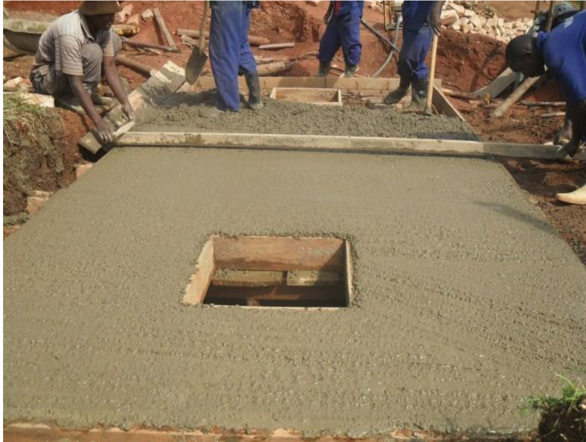
Top RCC with Opening for Manhole
