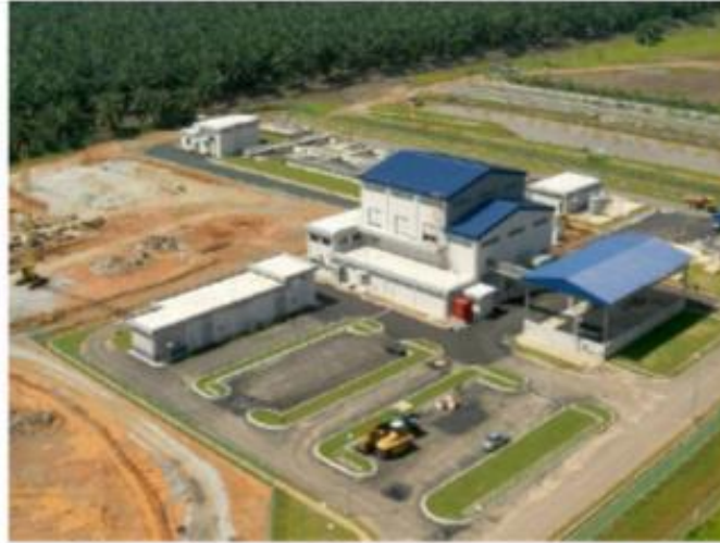
Centralised Sludge Treatment Facility
