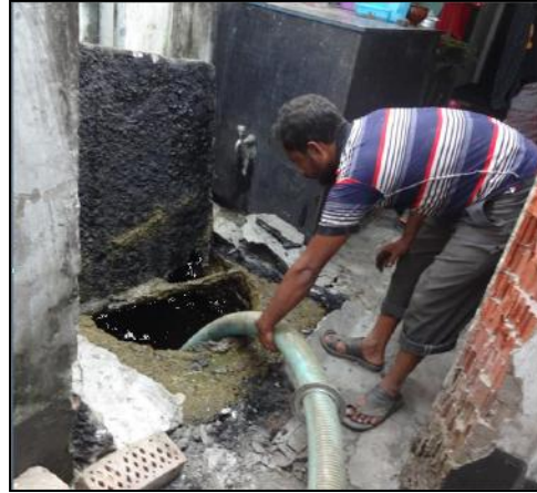
Emptying by vacuum pump (< 100 m sucking pipe) and truck
