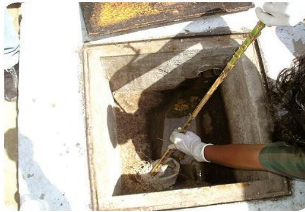
Removal of obstacle from the sewer pipeline
