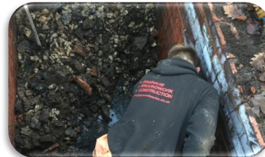
Cleaning and replacement of filter material
