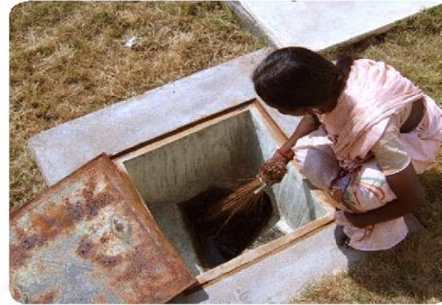
Cleaning of inspection chambers
