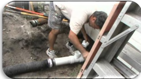
Replacement of pipes
