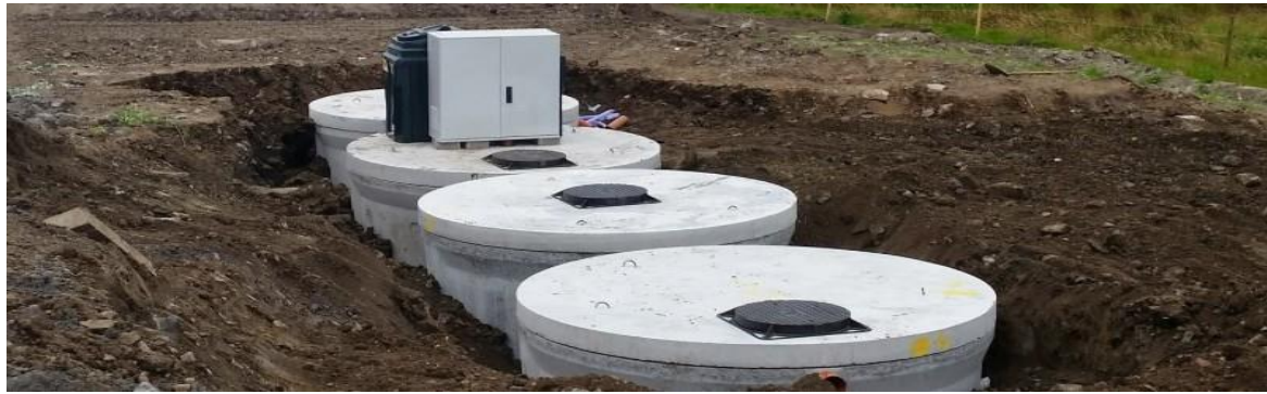
Figure 7.3: Septic Tank Riser
